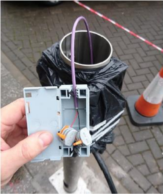
Figure 3 - Wago or Lever style connectors
