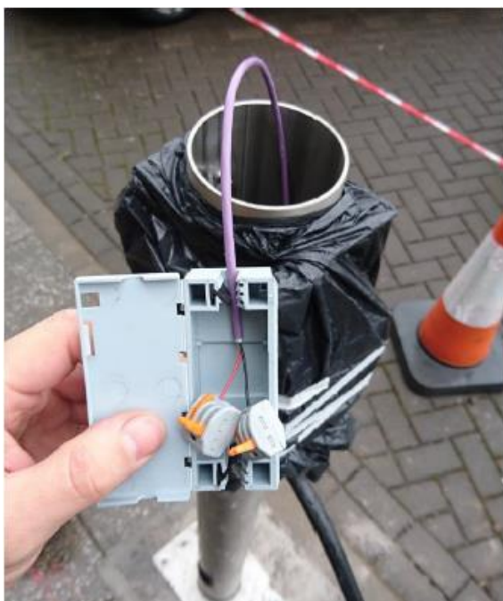
Figure 2 - Wago connectors linking up the serial bus
