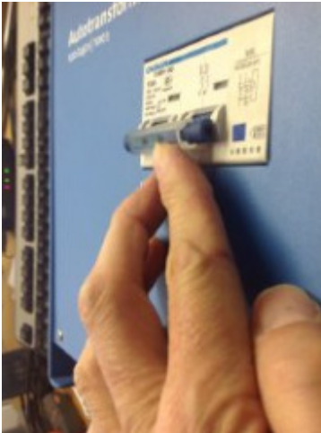
Switch the MCB to "ON"
