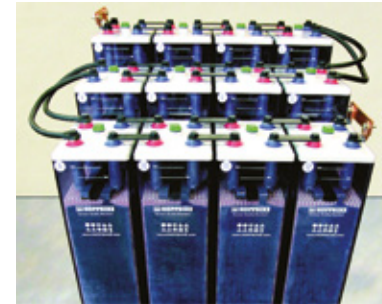
Fig. 5-16: Using row connectors and step connectors
