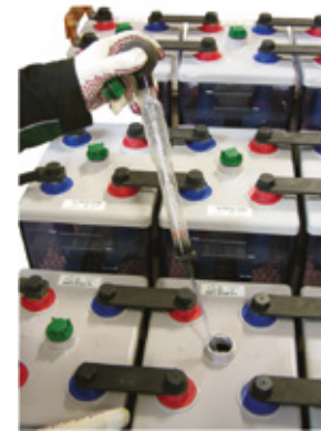
Fig. 6-2: Hydrometer
